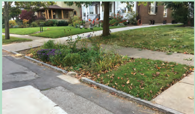
Curb inlets and rain gardens on Windsor Avenue. Fig. 083
