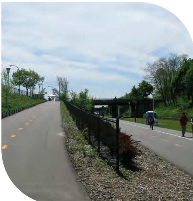
Example of an ADA approved, graded slope providing accessible transition for bicycle and pedestrian access between trail and park areas.
