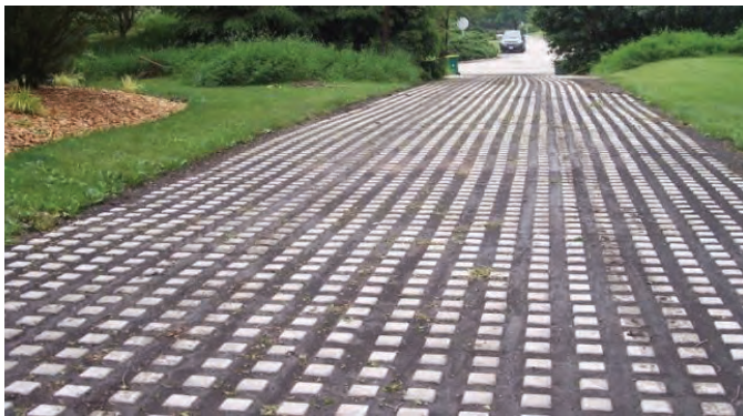
Example of a typical permeable paver system used for higher run off infiltration. Fig. 086 | (Reading Rock, n.d.)
