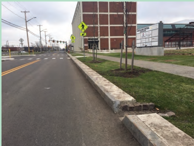
Curb inlets and trees on Northland Avenue. Fig. 084
