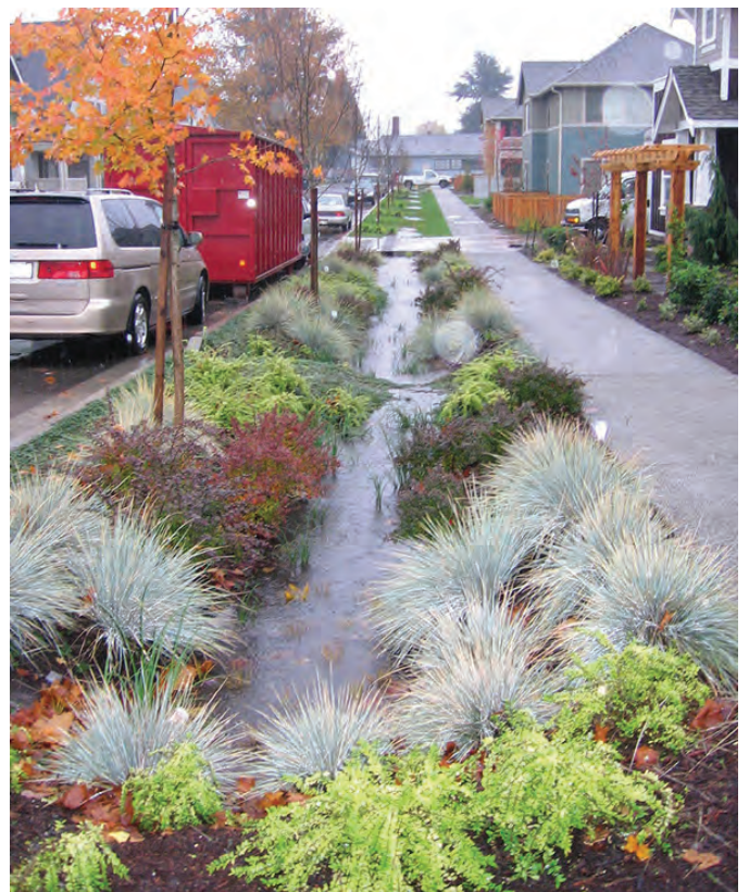
Example of a typical street scale, side walk adjacent Bioswale. Fig. 088 | (Tip of the Mitt Watershed Council, n.d.)
