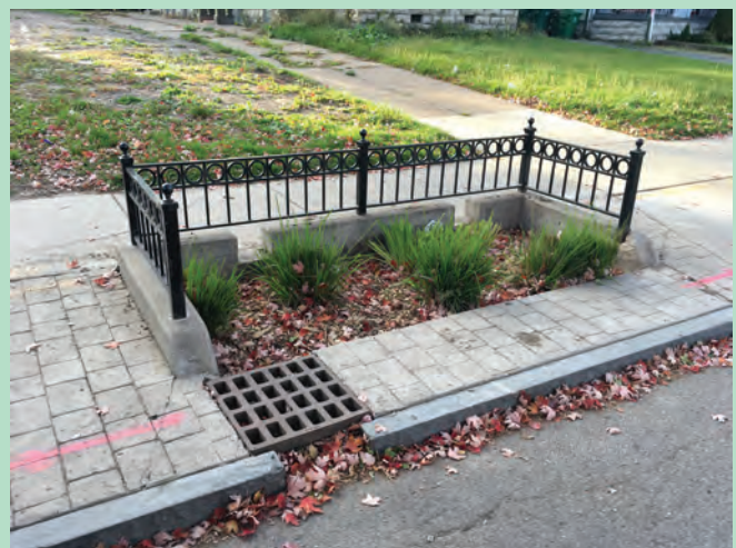
Curb inlets, rain gardens, and porous sidewalks on Elmwood Avenue. Fig. 085
