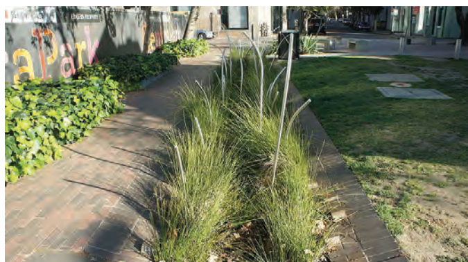
Example of a brick laid dry swale with native grasses and path lighting. Fig. 089a | (Wikimedia, n.d.)
