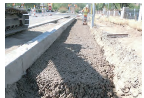
Compaction of CU-Structural Soil® during installation. Fig. 114 | Bassuk et al., 2015
