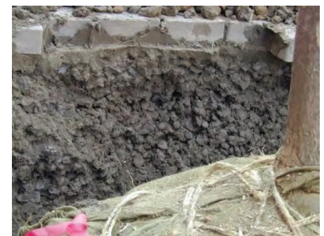
Closeup of CU-Structural Soil® after installation Fig. 113 | Bassuk et al., 2015
